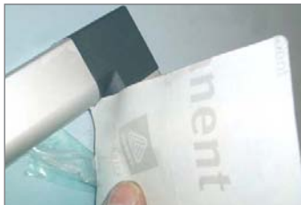
Fig. 5: any silicon residues are removed by sanding.
