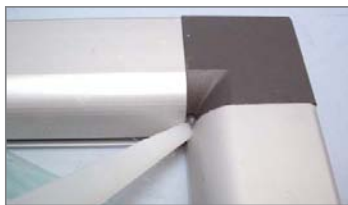
Fig. 4: the gap is sealed with silicon.
