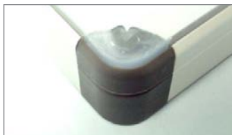
Fig. 10: looking at the outside corner of the framework, you can see how neat the joint is after siliconging.
