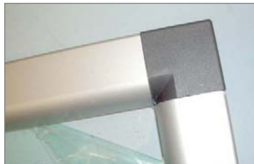
Fig. 6: view of the frame angle after sealing the gap with silicon.
