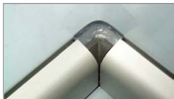
Fig. 9: the gap is sealed with silicon (inside of the framework).
